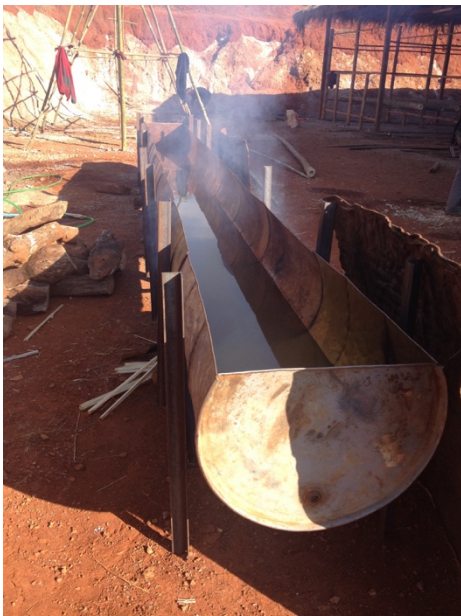
Solution heating in tank
